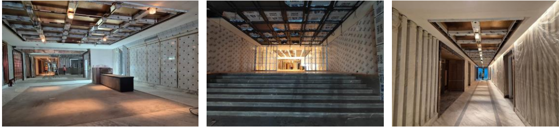
Note: Under construction images
