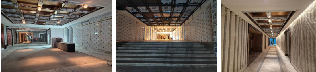
Note: Under construction images
